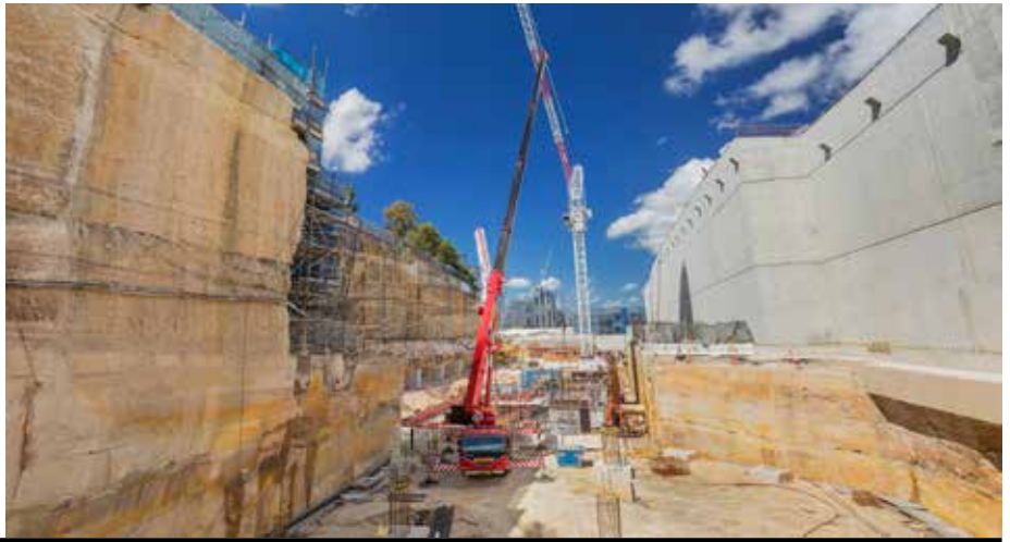
> Headland Park cultural space under construction, March 2014.
