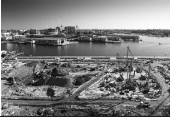
✓ Construction at Barangaroo South
