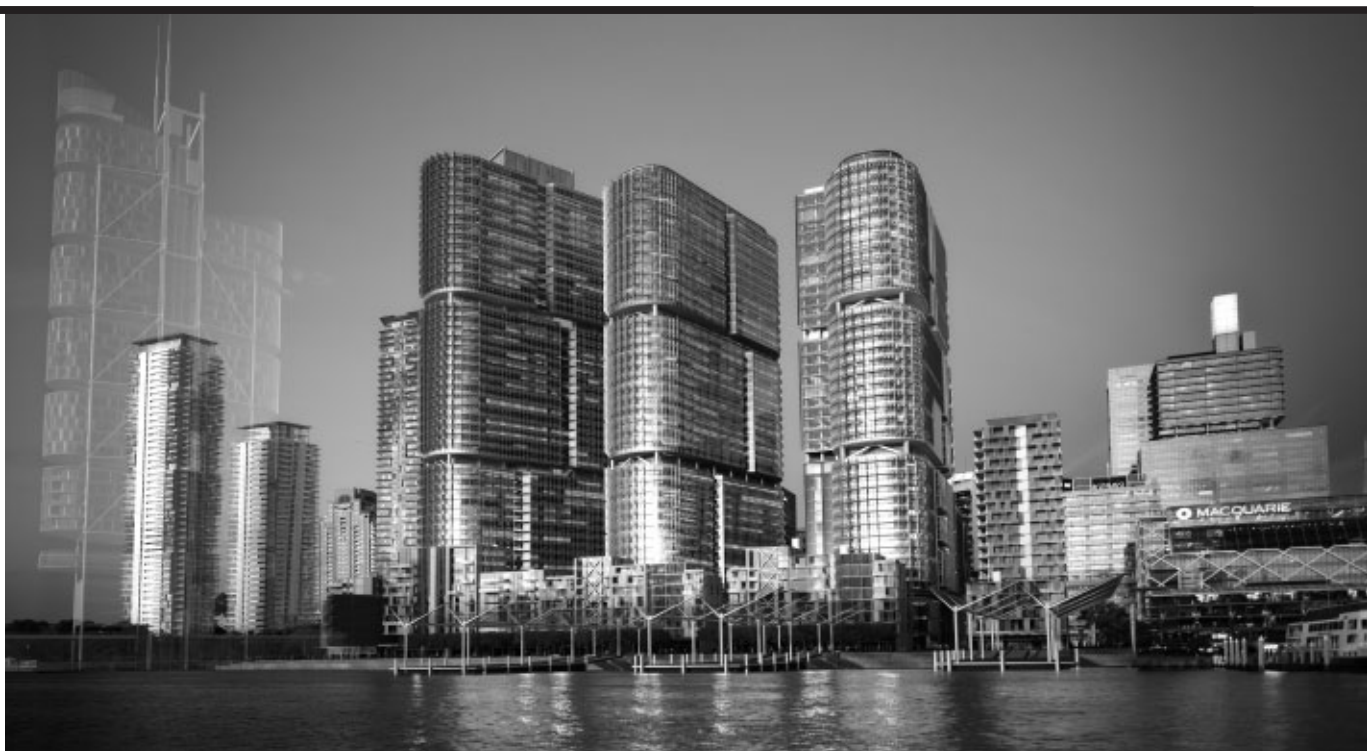
Commercial Towers at Barangaroo South
