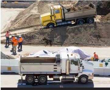
< Bulk earthworks and associated management of potential impacts such as dust.
