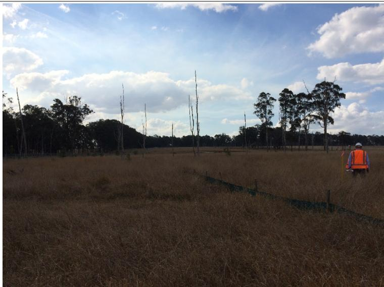
**Plate 3.5** Transmission corridor (view to north) – dead trees will be removed. Trees to the right are outside the easement (yellow star picket) and will be retained.
