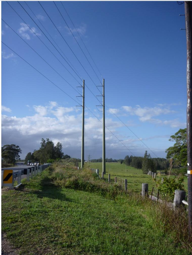
**Plate 3.8 Typical two-pole structure used at angles or changes in direction**
