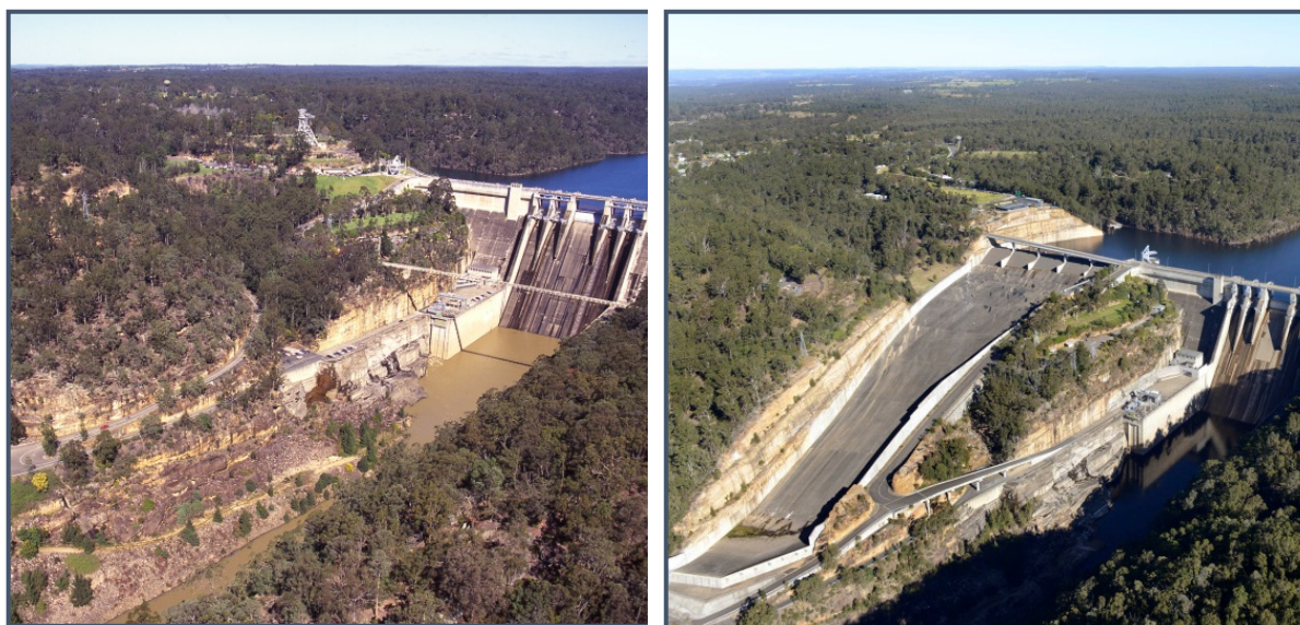
Figure 1.8 Warragamba Dam before and after construction of the auxiliary spillway
