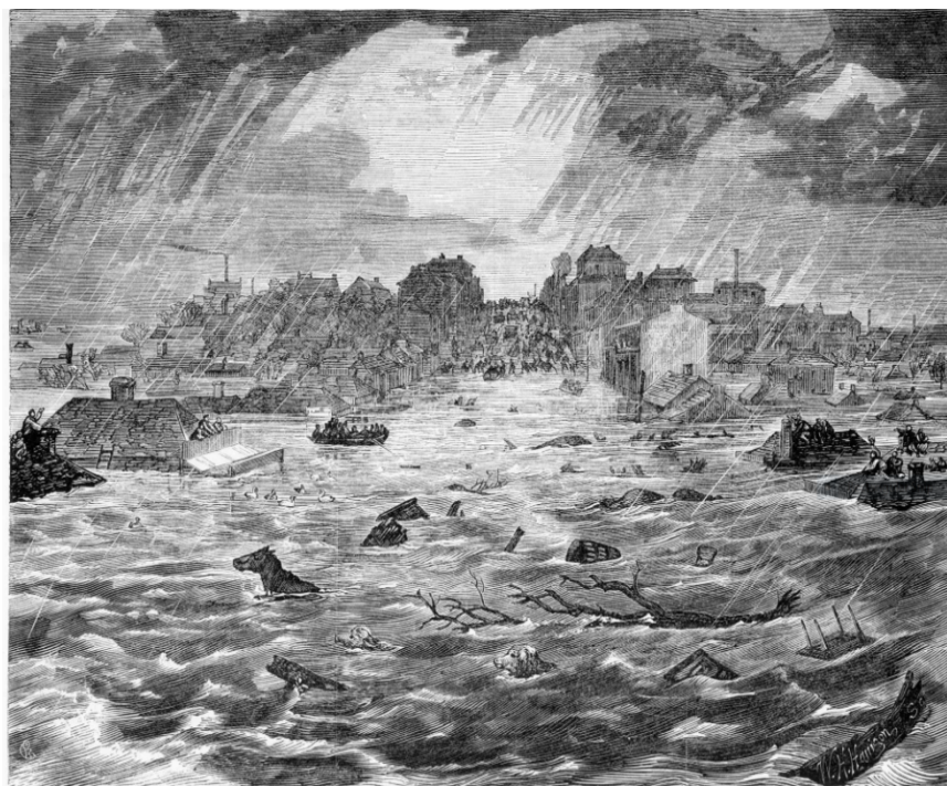
View of the Windsor 'island' in the 1867 flood
