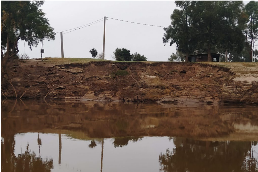
Rotational slip, straight reach, Pitt Town Bottoms, 3 April 2021
