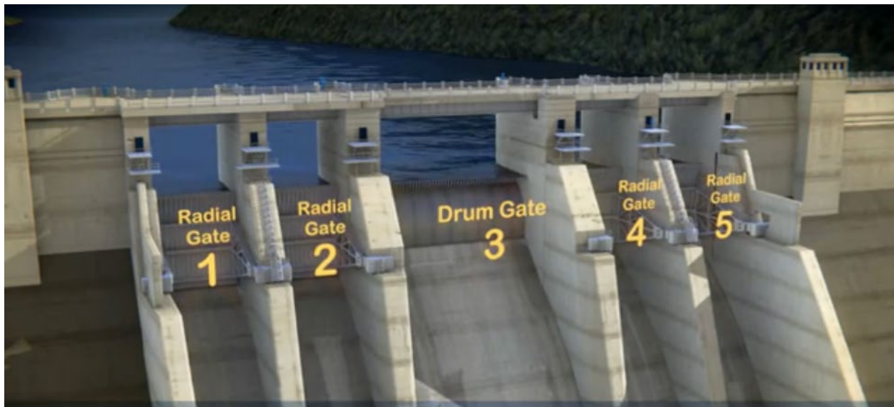
Figure F1. Warragamba Dam central spillway drum and radial gates
