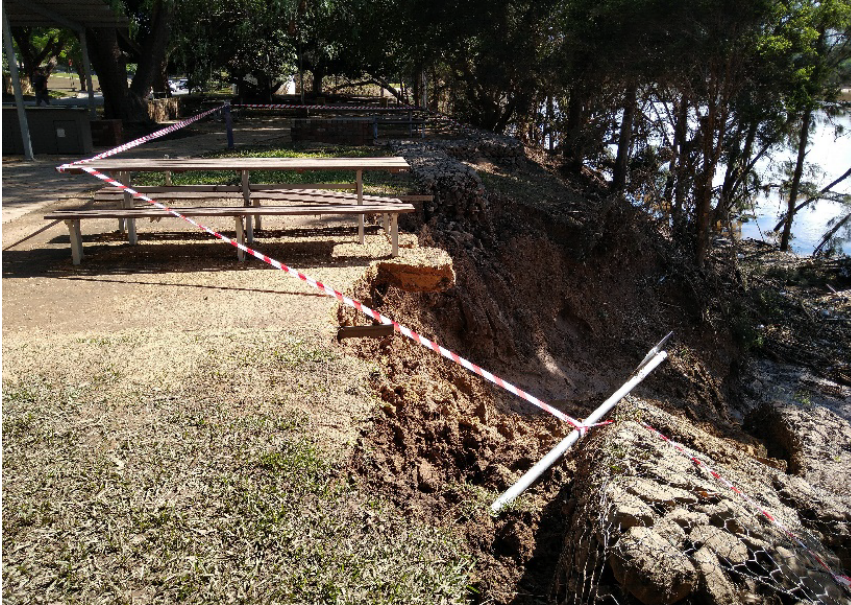
Collapsed rock gabions adjacent to The Terrace, Windsor
