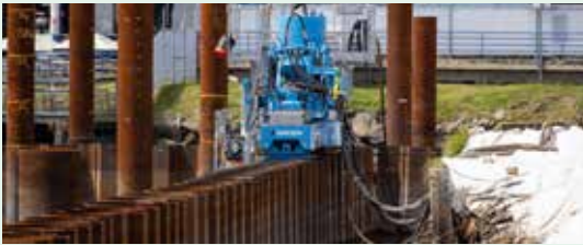
^ Cofferdam works on site
