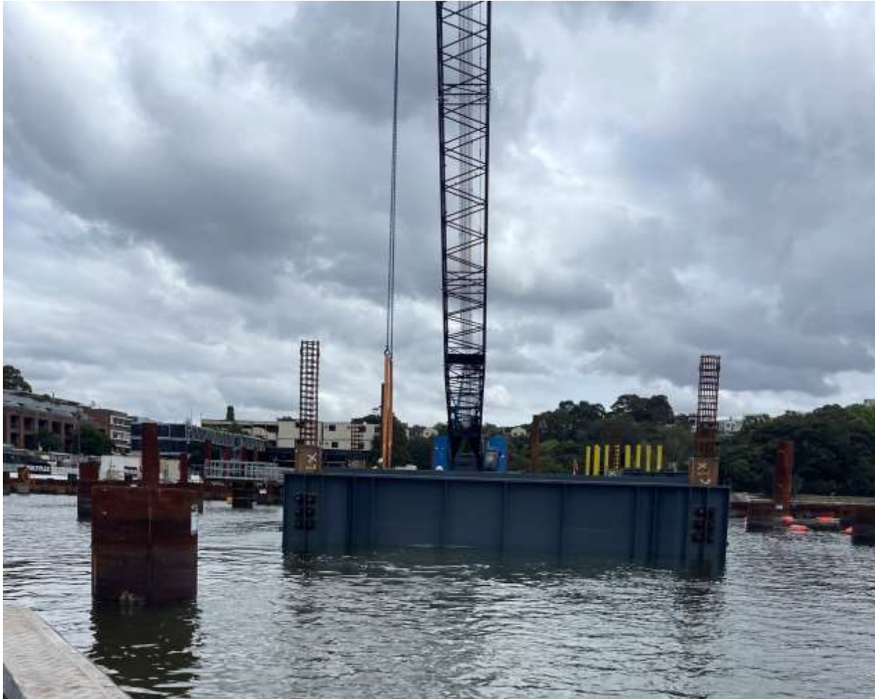
Tower crane column installation
