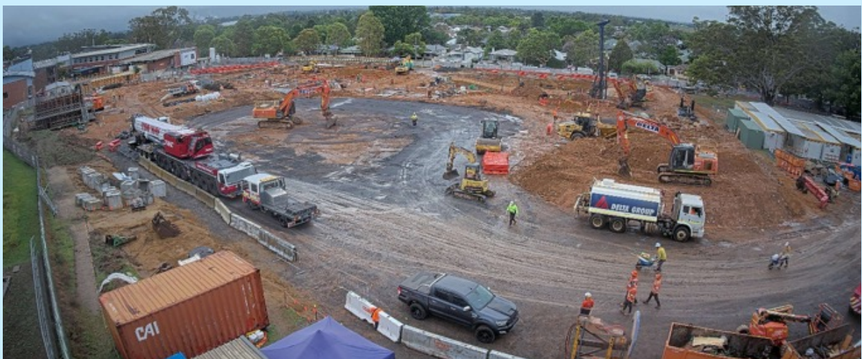
Aerial view of the Shoalhaven Hospital construction site
