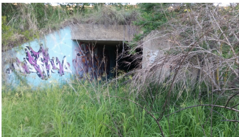
Photo 2. Western box culvert – M4
