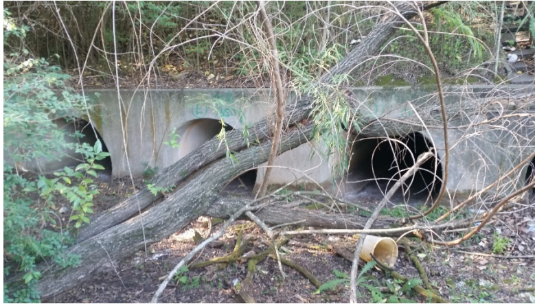
Photo 3. Western culverts – M4
