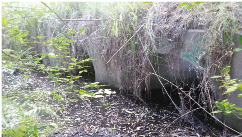
Photo 1. Eastern culverts – M4
