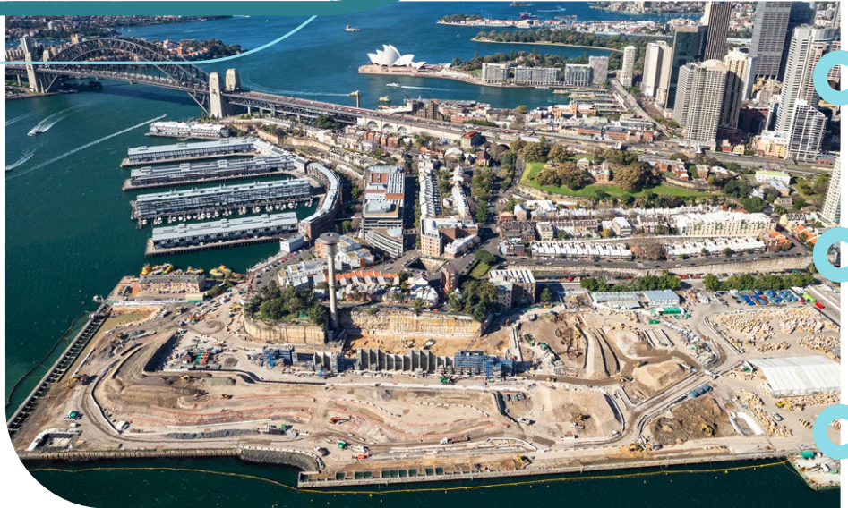
Above: Barangaroo Reserve and the Cutaway under construction
